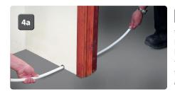
When floor heating pipes need to pass through walls, drill the holes before laying and fixing boards to prevent any damage to the boards. Protect and seal the pipe ends with tape. To prevent kinking, one person should feed the pipe through the hole whilst another draws the pipe through from the other side, it is a good idea to use pipe conduit to run through walls (4a).
