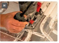
Using a router with bit set to 16/12mm depth depending on pipe, gently cut the new channel following the marker pen layout **(H)**. Ensure the channel is clear and free from debris, if required the channel can be lined with aluminium tape. Lining with aluminium tape is not required in areas with highly concentrated/close floor heating pipes.
