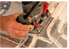
Using a router with bit set to 16/12mm depth depending on pipe, gently cut the new channel following the marker pen layout **(H)**. Ensure the channel is clear and free from debris, if required the channel can be lined with aluminium tape. Lining with aluminium tape is not required in areas with highly concentrated/close floor heating pipe.
