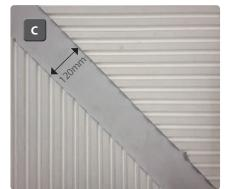
Extra pipe channels can easily be cut using a suitable router and bit. In order that a smooth bend is formed, lay and shape the pipe onto the area where the channel is required, gently bending the pipe to follow a gentle curve. Once the lay of pipe has been established, follow the curve with a marker pen, marking directly onto the board the route to be routed **(F/G)**.
