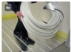
This will help deter the pipe from trying to twist and keep tension pointing downwards, ease the pipe around and into the bend. Lay the pipe into the return or corner, gently forming and pushing the pipe into the channel as it works around the bend (9d/e).
