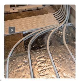
Do not push the 45° cut edges up against each other, leave a gap approximately 120mm wide **(C)** this will allow the pipe to be formed and bent as it changes direction from one straight channel to another. Take care not to form to tight a bend and kink the pipe.
